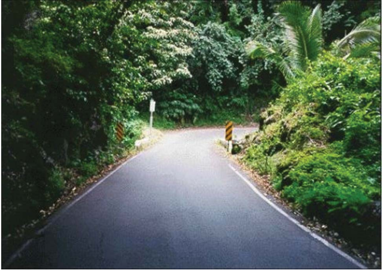
Figure 43. Hāna Belt Road near Waiele Bridge, illustrating the narrow roadway tightly encroached upon by bedrock ridges and jungle vegetation (Wilson Okamoto & Associates 2001)
