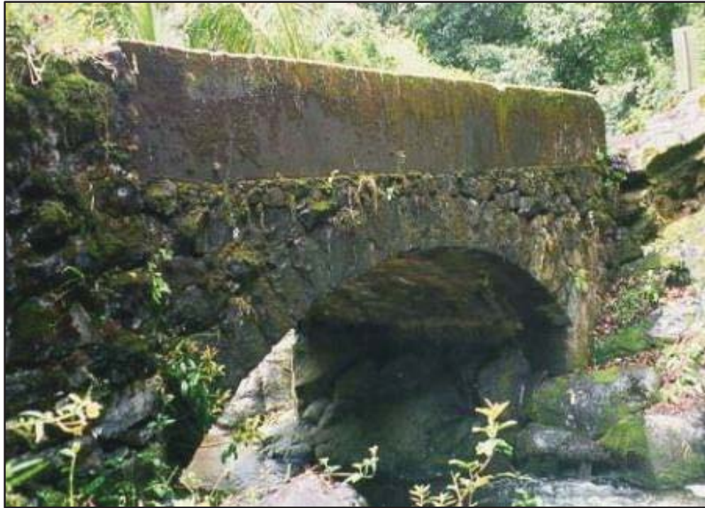
Figure 41. Hāhālawe Bridge, a characteristic masonry arch style bridge (Wilson Okamoto & Associates 2001)
