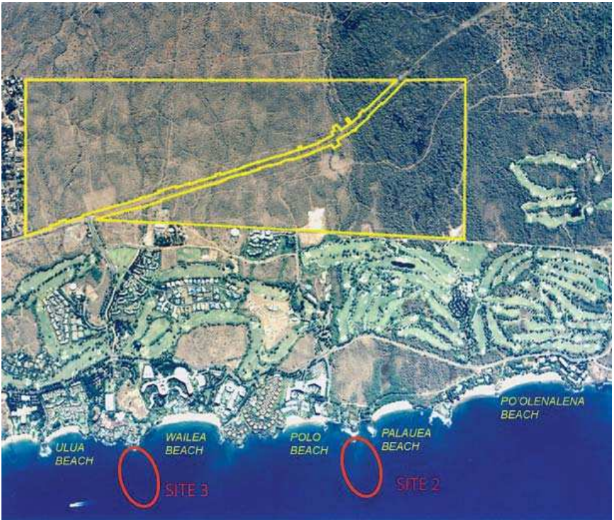
FIGURE 1. Aerial photograph of Wailea Maui coastline showing locations of beaches downslope from Wailea Golf Courses and Honua`ula project site (outlined in yellow). Locations of representative marine biota sampling sites are shown as red ovals. Site 1, which is considered a control station, is located within the `Ahihi-Kina`u Natural Area Reserve, approximately 4 km south of the Honua`ula project site.
