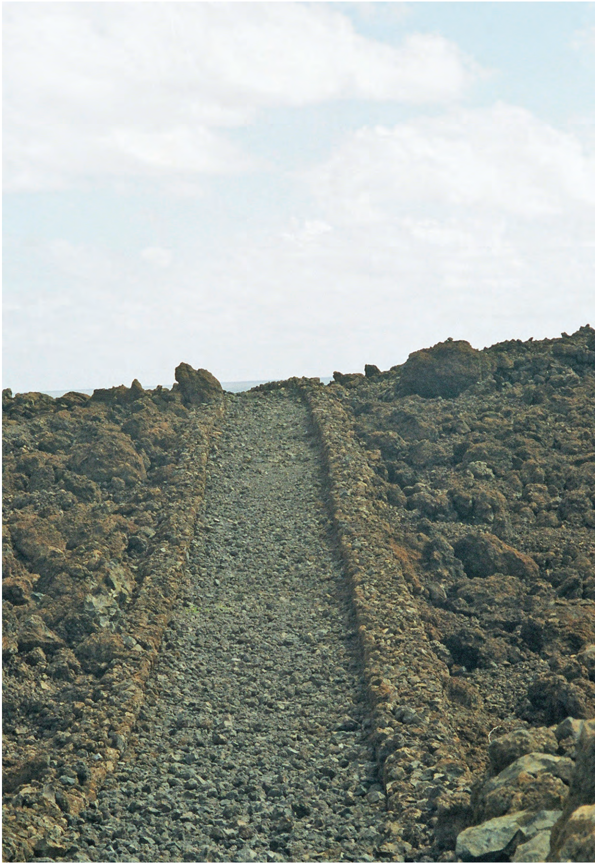
FIGURE 28 SECTION OF HOAPILI TRAIL (C. 1824-1834) BUILT UNDER GOV HOAPILI AS A HORSE AND CART ROUTE OVER THE LANDS OF KULA, HONUA'ULA, KAHIKINUI AND KAUPŌ.2002.
